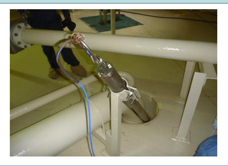
E Exia Intrinsically safe Labkotec 2 wire WBS 3000 Water sensor
